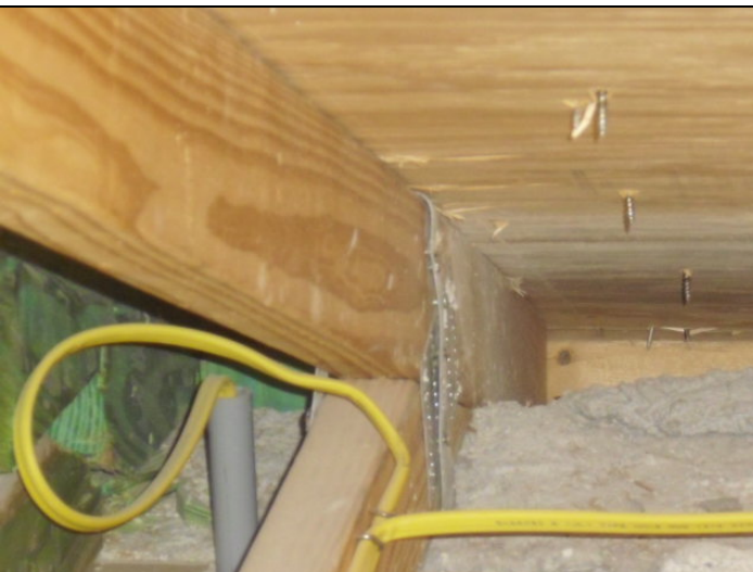
Roof to wall attachment
