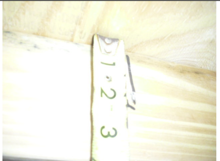
Roof deck attachment
