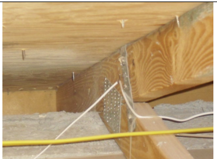
Roof to wall attachment
